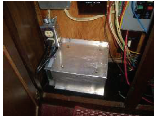
The new WFCO fuse panel
